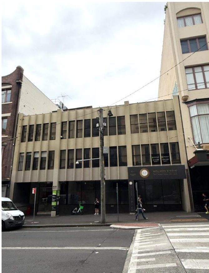
Figure 2: Site viewed from Bay Street, looking east
