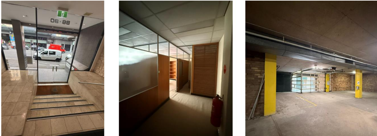
Figure 5: Ground level foyer, remnant original offices and basement parking area
