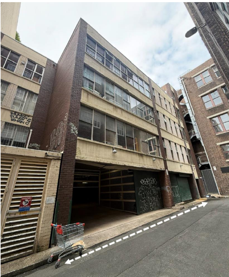
Figure 4: Site (dashed line) viewed from St Barnabus Street, looking south-west
